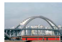
Lupo bridge, Shanghai
